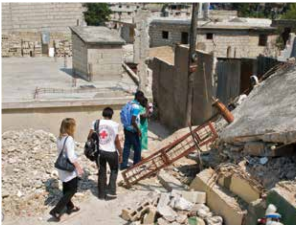
Figure 4. An ICRC and Haitian Red Cross Team survey damage after the Haiti Earthquake. (ICRC)
